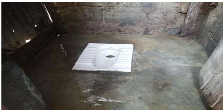
Figure 13: A slab toilet constructed within proximity of target households in Mukuru
