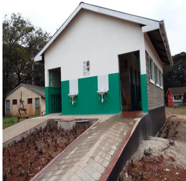
Figure 11: Boys toilet block constructed by ChildFund at Kasarani Primary School
